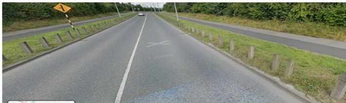
Bollards along the Naas Southern Ring
