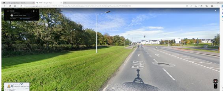
Another example of a mounded grass verge is opposite the main entrance into the Pipers Hill Campus. Below.
